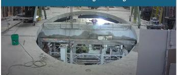
An ellipse opening was a renovation to the existing slab of a corridor to create an opening to the lower level at the Minneapolis Airport. The ellipse was carefully cut using a variety of different saws to finish off the precise cut.
